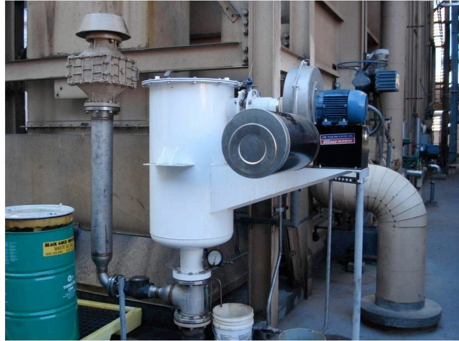
After – Solberg “BAE” Blower Assisted Oil Mist Eliminator
